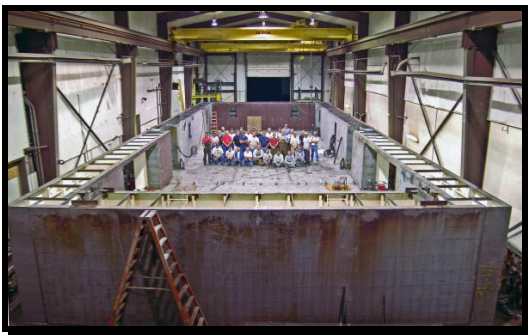
Lower Section of Truck Dump Hopper for Coal
