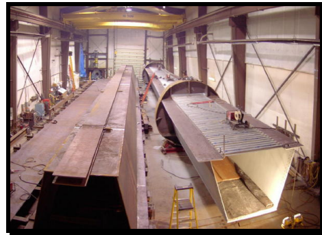
Bridge Tub Girders For Alaska Bridge
